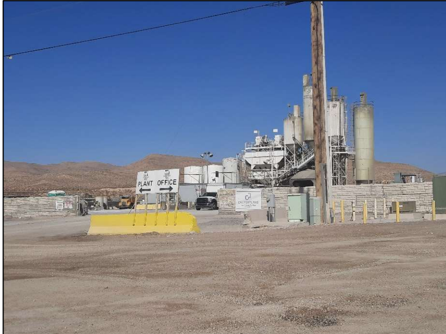
17400_American Eagle Ready Mix Plant 2 Sloan - 1.jpeg
