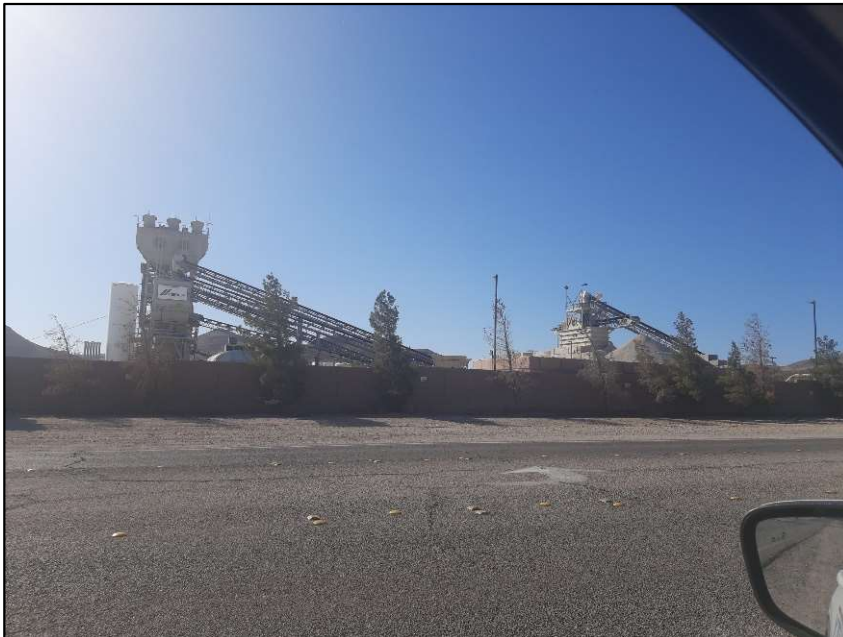
15914_CEMEX Construction Sloan- 2.jpeg
