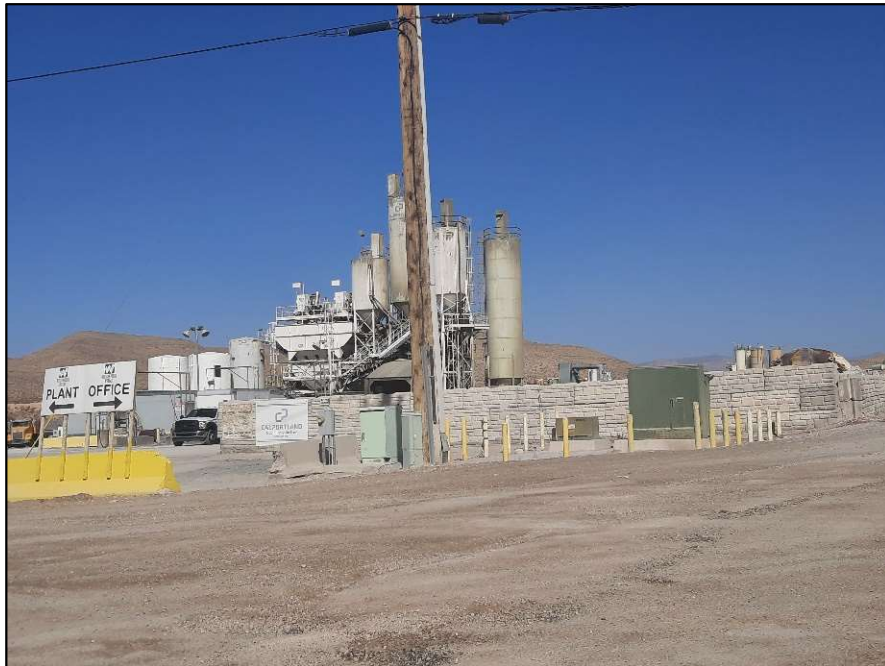
17400_American Eagle Ready Mix Plant 2 Sloan - 2.jpeg
