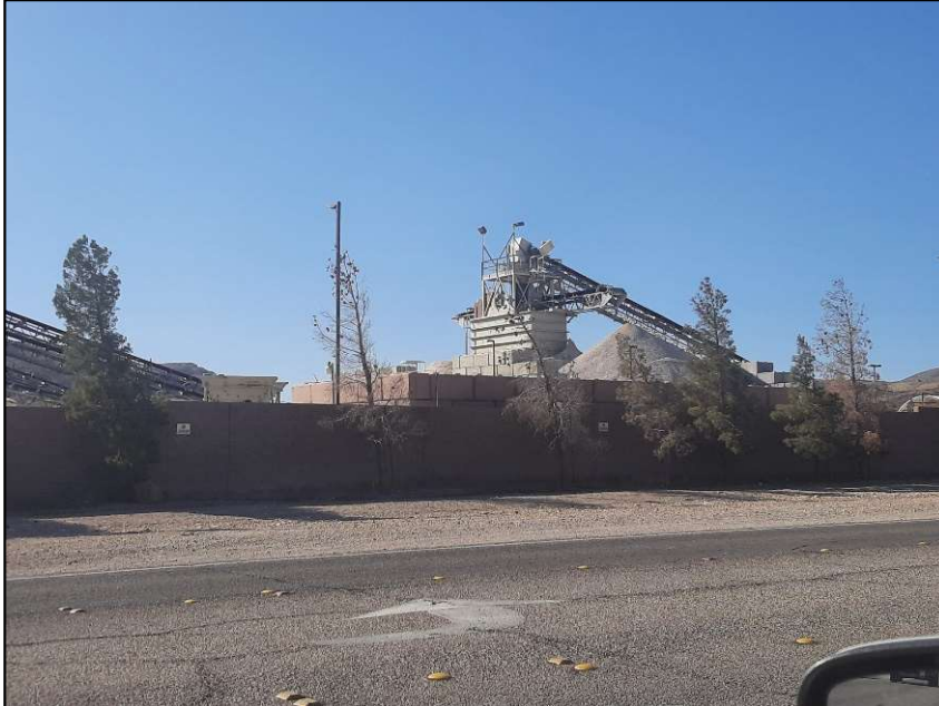
15914_CEMEX Construction Sloan- 1.jpeg
